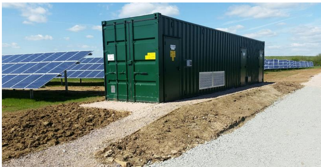
Plate 4: Typical Unit Housing the Transformers and Switchgear
